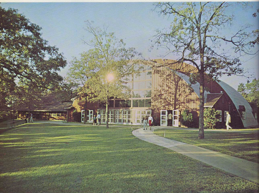
Reflected light from Dining Hall windows creates a striking scene. The Dining Hall building houses student lounge facilities and some class areas in addition to its kitchen and dining rooms.
