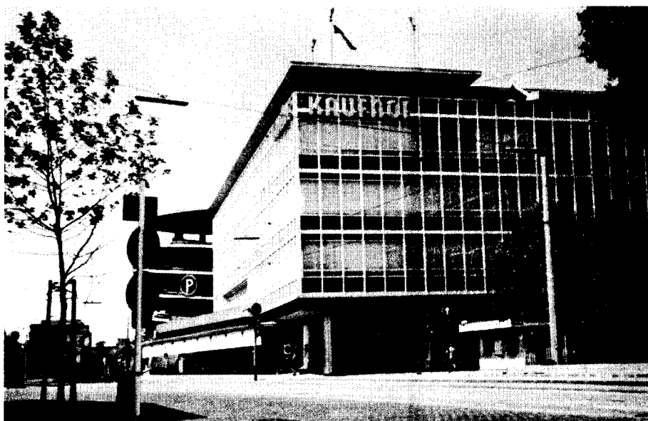
From the ruins of Köln rises this new Department Store. At left in rear, marked with the letter "P", for parking, is a modern circular ramp leading to a 5-storied indoor parking building.
