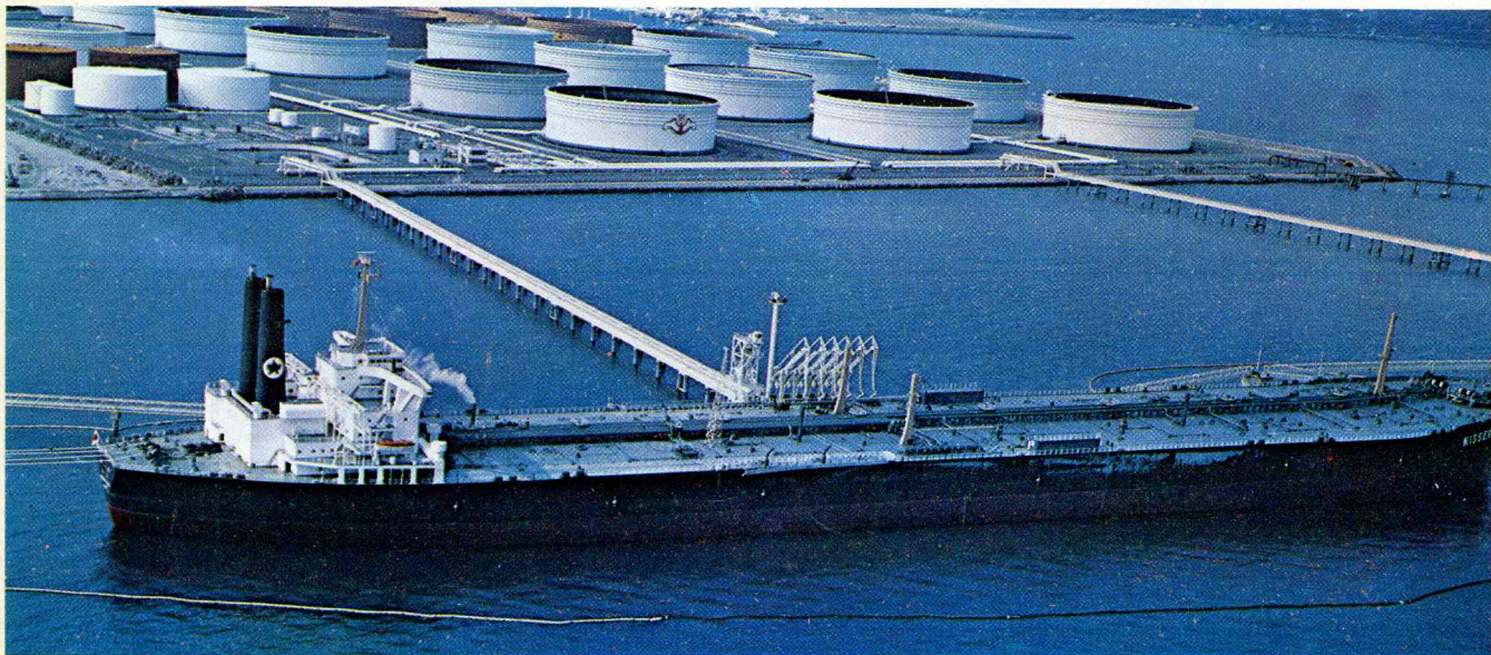
ONE OF THE WORLD'S LARGEST TANKERS , the 372,698 DWT Nisseki Maru , at Kiire Terminal. Located in Kogoshima Bay, Japan, the terminal is currently equipped with 12 oil storage tanks to hold petroleum shipped from Middle East.
