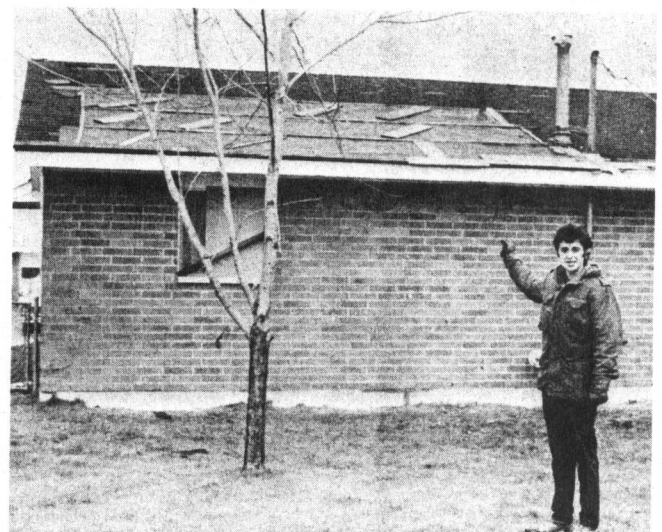
PROOF OF PROTECTION — Only four houses away, tornadoes cut a swath, leveling the area, but here Dayton member Steve Wyke points out his home was virtually untouched except for some missing shingles and a few broken windows. (Photo by Mark Robinson)
