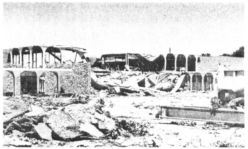
TWISTER'S DAMAGE — One of the tornadoes which hit Tulsa June 8 caused extensive damage to Oral Roberts University in the southern part of town. The Oral Roberts Association Building and the Aerobics Building, which was under construction, were both destroyed. An estimated $1 million damage was caused to the institution. [Photo by Phil Edwards]
