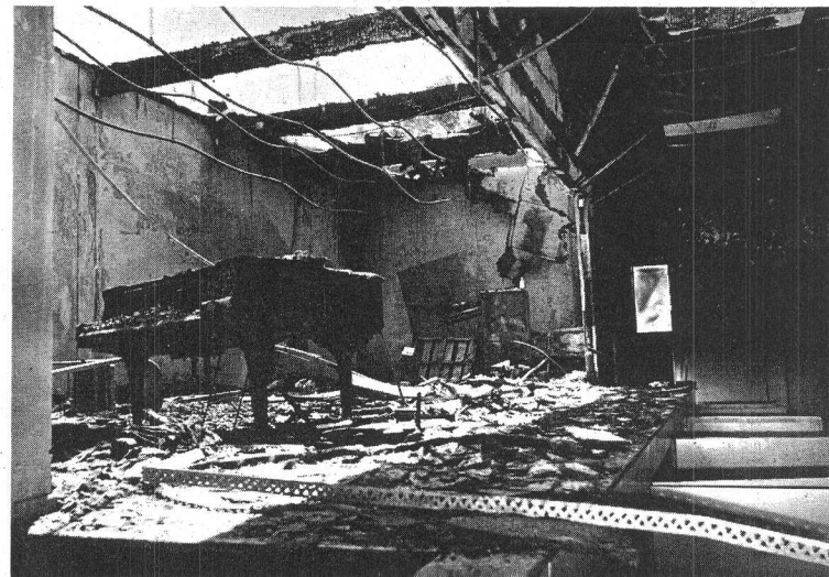
FIRE HITS CHURCH HALL — The Church-owned building in which the Norwalk, Calif., churches were meeting was gutted July 25, causing an estimated $75,000 damage. Police suspect arson. The hall had been the target of vandalism before the fire. The churches are meeting temporarily in the Ambassador Auditorium on the nearby Pasadena campus until a new meeting place is found. [Photo by Ken Evans]
