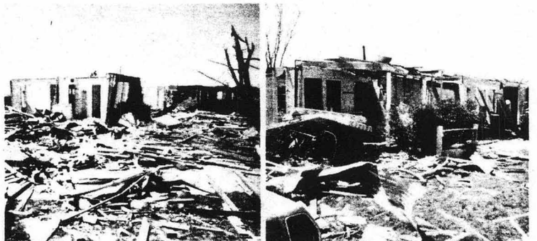
TORNADO DAMAGE — The homes of several members were among those heavily damaged and destroyed by tornadoes that swept through Wichita Falls, Tex., April 10. Shown above are the homes of Mrs. F.E. Chadwell, left, and Mr. and Mrs. Jaime Calderon of Wichita Falls. Only portions of the walls were left in either house. (Photos by David Carley)
